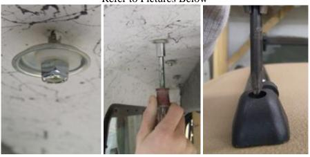
9. After all the screws are tightened use vise-grip type pliers to hold the end of the screws and move them back & forth until they snap. (These are break-away type screws. Notice some screws may have to be filed or ground down if they do not snap)
